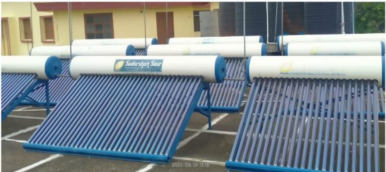
Rooftop Solar Water Heaters
