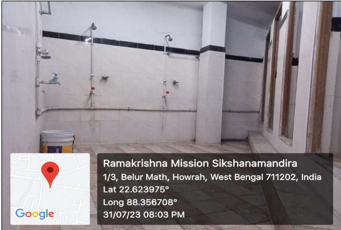
Hostel building has large toilet sections for the trainees
