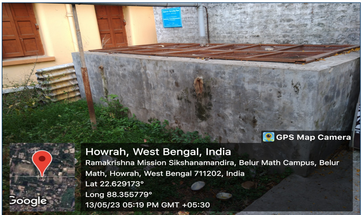
Water Reservoir near the main gate of the college
