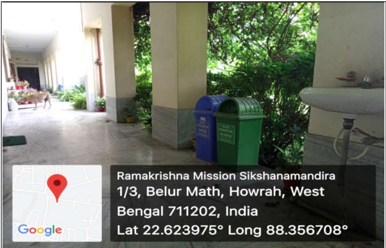
Bins placed at the ground floor of college verandah
