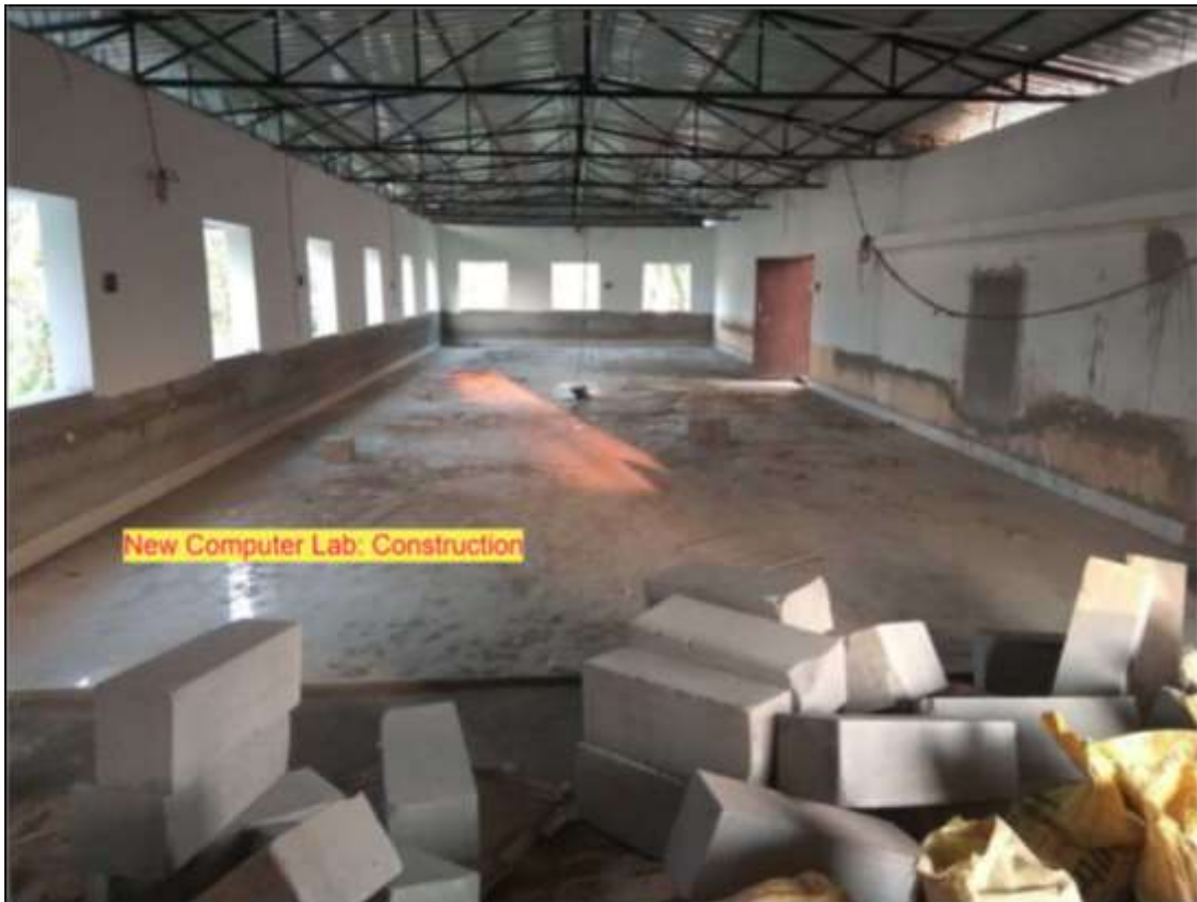
Construction of Multipurpose Computer Lab
