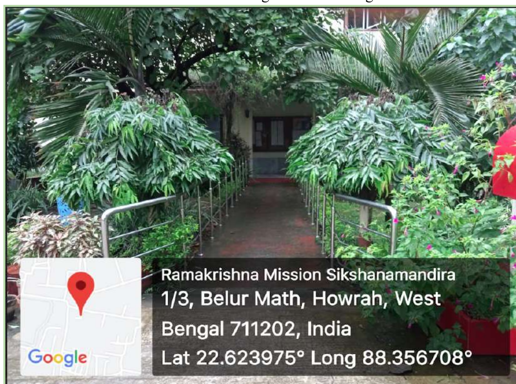
Ramp Facility at the college building
